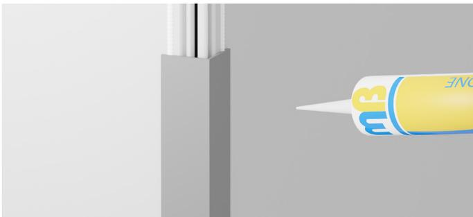
Once all panels have been fitted, any external angle trims can be installed around window enclosures or fitted around any pipework which has been boxed in using a silicone adhesive.
