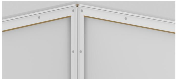
Once the bath has been sealed, trims should be fitted using screws or staples. If you are unable to fit trims with screws or staples, a silicone based adhesive should be used and allowed to cure before fitting any PVC panels.
