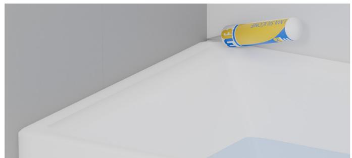
If applicable, fill your bath tub with water prior to sealing. This weighs the bath down during the sealing process. Once sealed, silicone should be allowed to fully cure before the bath can be emptied. This compresses the silicone and prevents splitting in the future.
